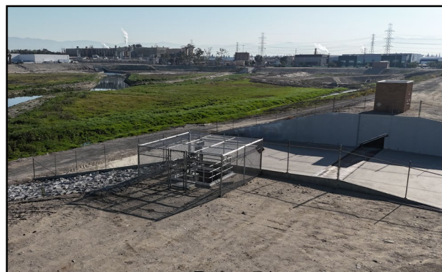
Outlet Control Gate/Rubber Dam System
